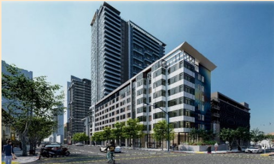
Kettner Crossing (64 units) 1590 Kettner Blvd San Diego, CA 92101
